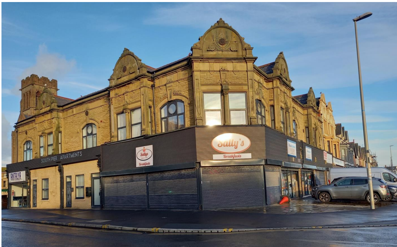
Locally listed former club, now apartments
