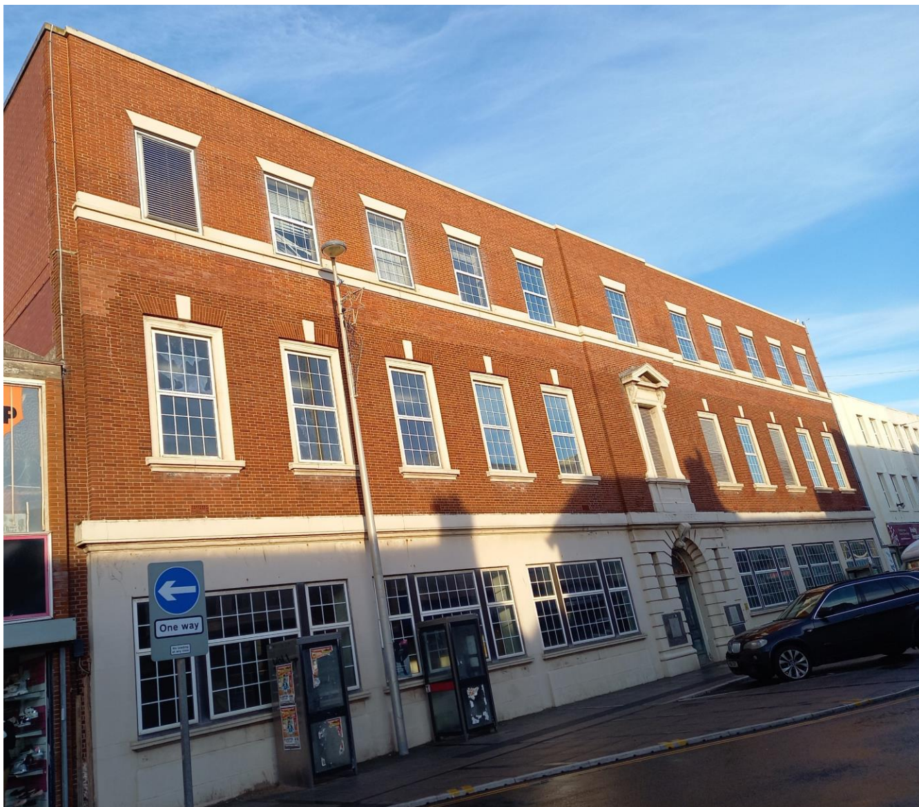
Locally listed former post office
